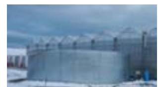
A tank with a rainwater utilization system
