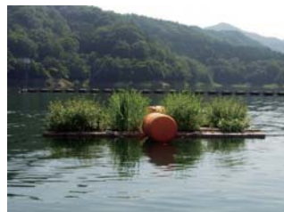
Ex. 1. Trial installation of floating-type samples of P-CON
