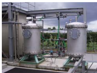
Ex. 4. Phosphorus-removal plant
